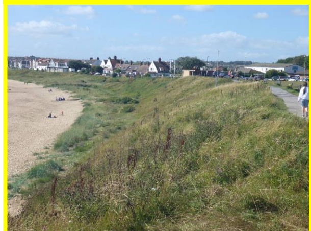
Generally stable cliffs with occasional small and localised slumps (/0601C01)
