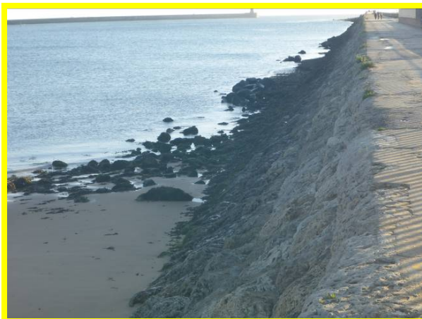
South Pier in overall fair condition along northern face, landward end(/0103C01)
