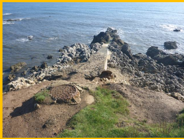
Outfall and manhole (/0401C04)
