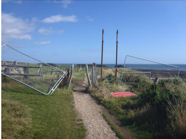
Fencing and signage blown over by the wind
