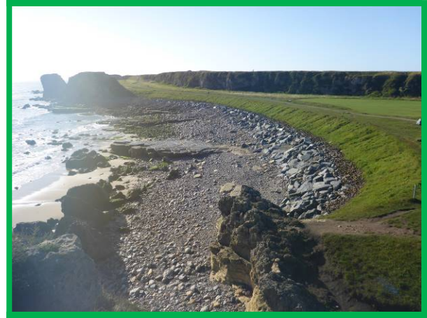
Rock revetment and re-graded slope at Graham's Sand (/0302C02)
