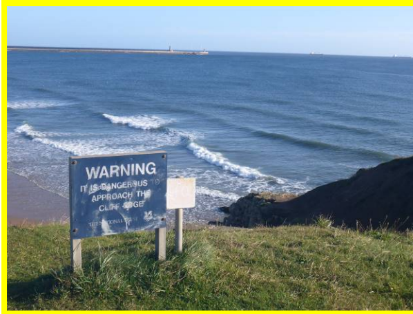
Localised slumps in soft material at Trow Point (/0302C01)
