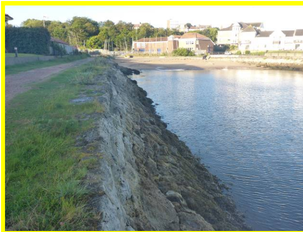
Grouted masonry revetment in fair condition (/0101C01)
