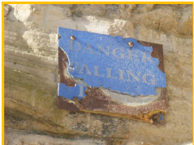
One small warning sign – broken condition (/0401C03)
