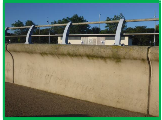
Littlehaven promenade and seawall in very good condition (/0102C02)
