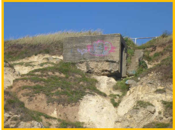
Pill box above access ramp (/0401C04)
