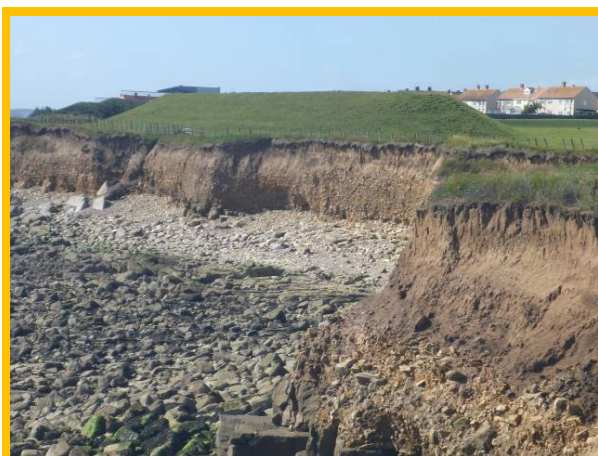
Regular small and localised slumps at southern section of Rifle Ranges (/0601C02)
