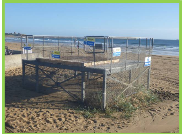
Disused lifeguard station platform next to reconstructed wall promontory (/0201C04)
