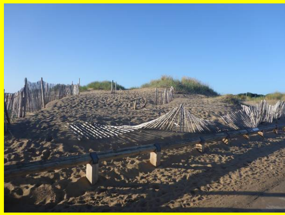
Fencing blown over (/0201C01)
